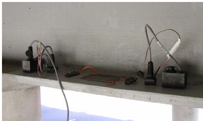
Figure 4.8: MicroSAFE Units Paired on Bridge
