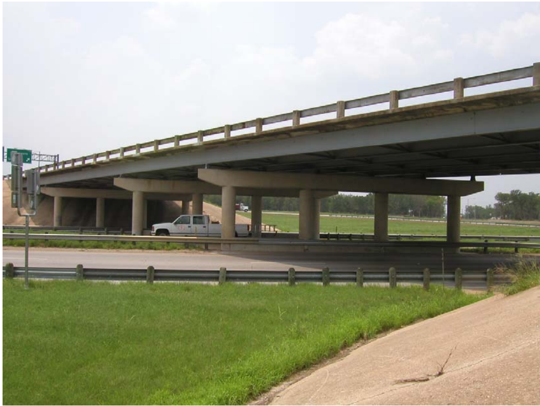
Figure 4.6: U.S. 183 / Texas 71 Overpass
