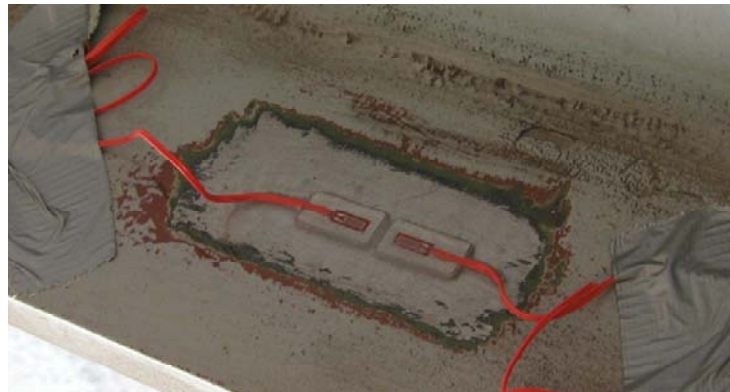
Figure 4.7: Paired Strain Gage Placement
